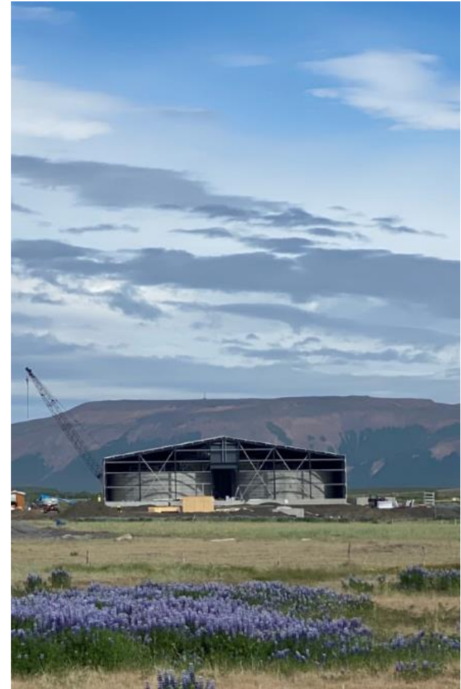
Picture taken at Kópasker just before house was finished in July.
